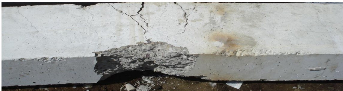
Figure (9) Crack pattern at failure for un-strengthened column C1.
