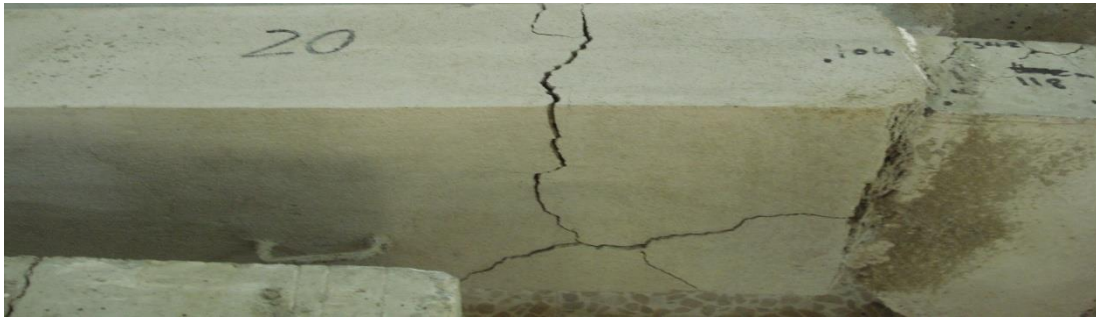
Figure (15) Crack pattern at failure for column C5 .
